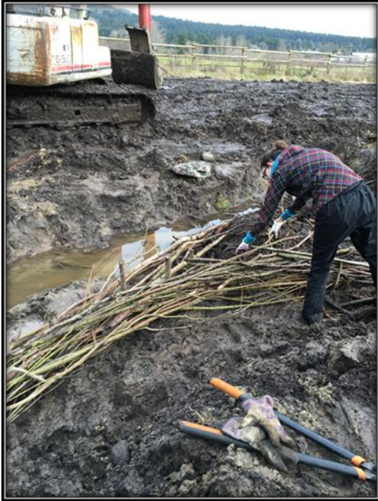
FIGURE 21. BUILDING A WATTLE ON THE SOUTH BANK.
