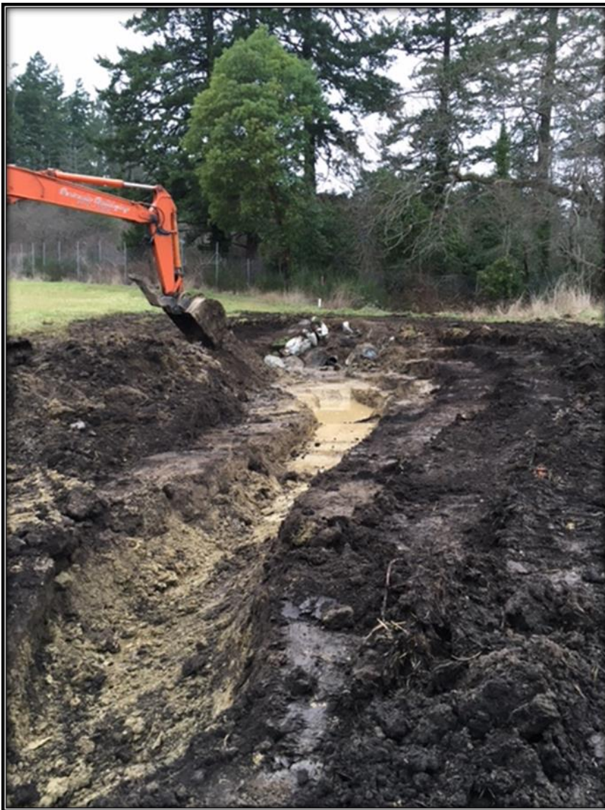
FIGURE 20. FIRST DAY OF RESHAPING ACCOMPLISHED BY MEANS OF AN EXCAVATOR.
