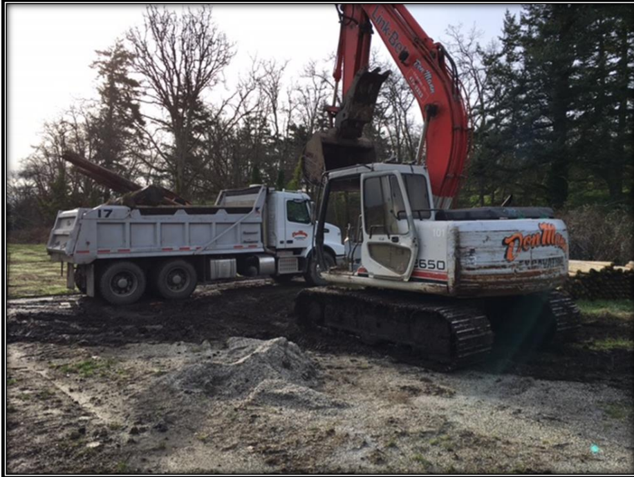
FIGURE 18. TANDEM AND EXCAVATOR USED IN THIS RESTORATION.
