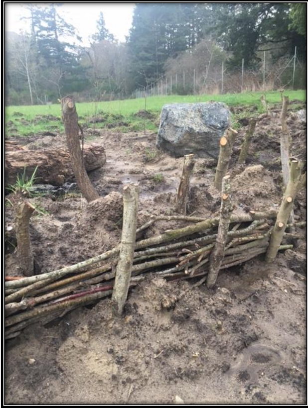
FIGURE 27. AFTER A HARD RAIN CLAY BEGAN TO OOZE UNDER AND THROUGH THE WATTLE.
