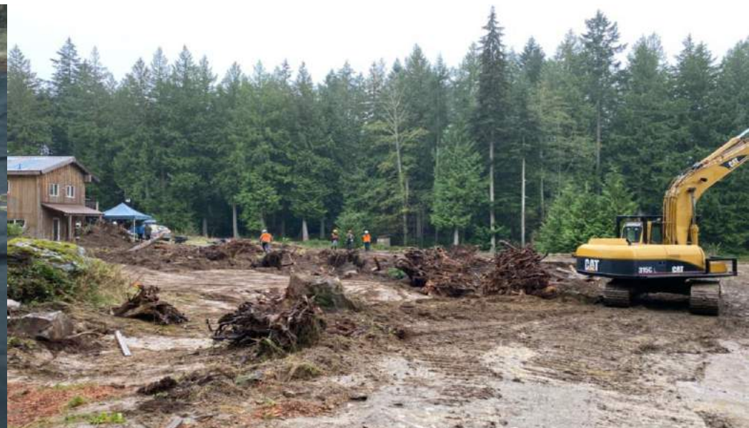
Upper right: excavator adds soil and habitat features such as stumps back into the wetland Lower right: volunteers bring a table to the “outdoor classroom” area on the wetland edge
