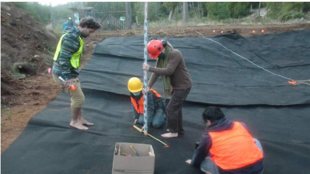
Upper left: marking points for pegging the liner Lower left: volunteers plant around the wetland. Note the use of burlap and cages.
