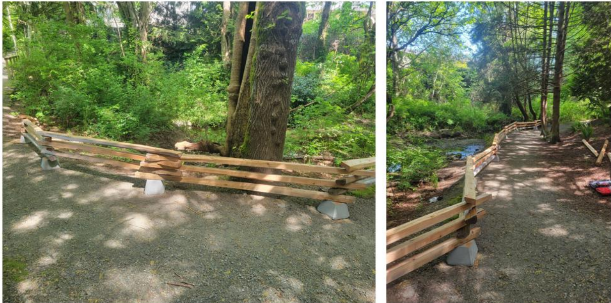
Figure 9. Newly installed split rail fence around the restored area (late April 2025).
