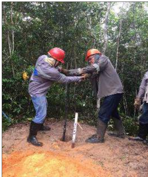
Picture 1. Auger drilling
