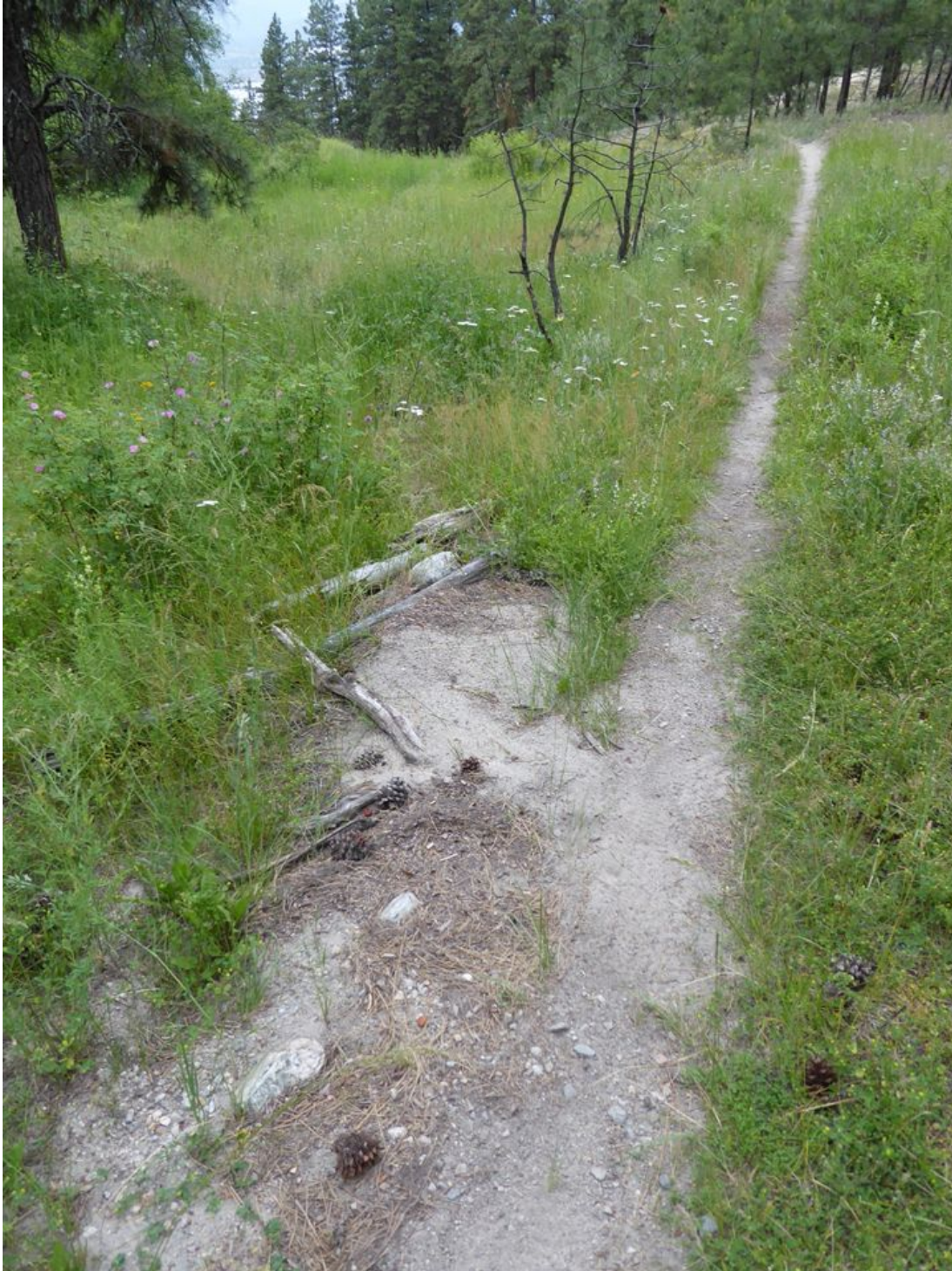
Figure 14. Junction between Chute Out and restored trail in June 2017. Note the thick vegetation cover along the restored trail tread. Also note the accumulation of sediment at the junction that was deposited following snow melt and spring rain storms. (Photo: T. Redding)
