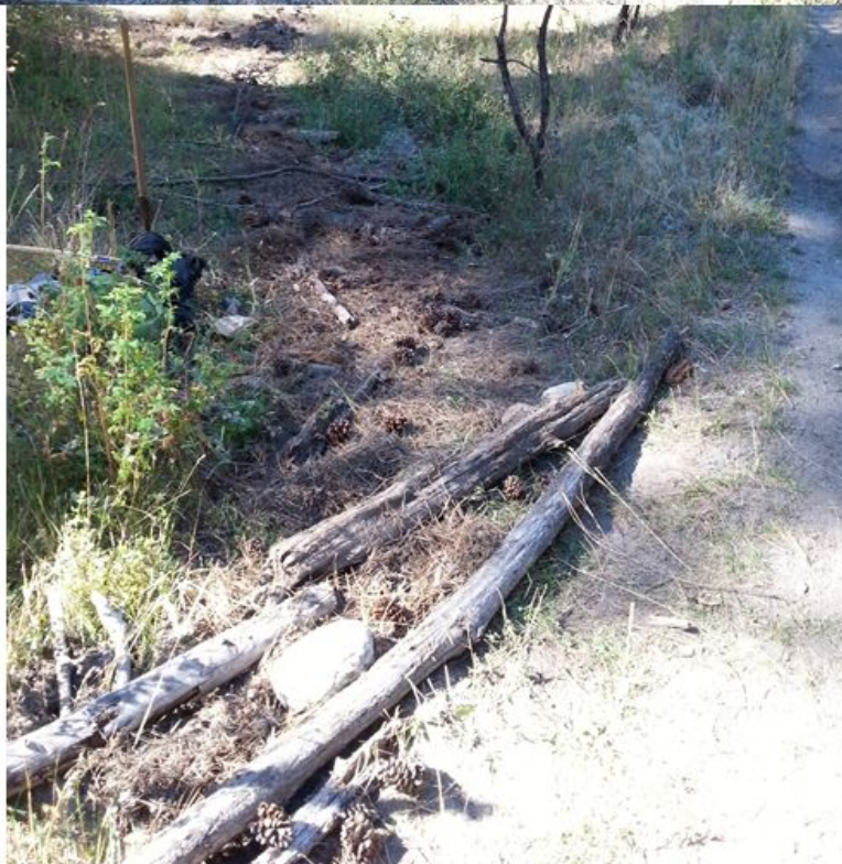
Figure 11. Junction between decommissioned and new segments of Chute Out. Upper photo shows intersection prior to restoration and the lower photo shows post-restoration treatment with organic material spread over the decompacted trail tread. In lower photo note the presence of logs and rocks to disguise and discourage use of the trail and capture and store any sediment running down Chute Out.. (Photos: T. Redding)
