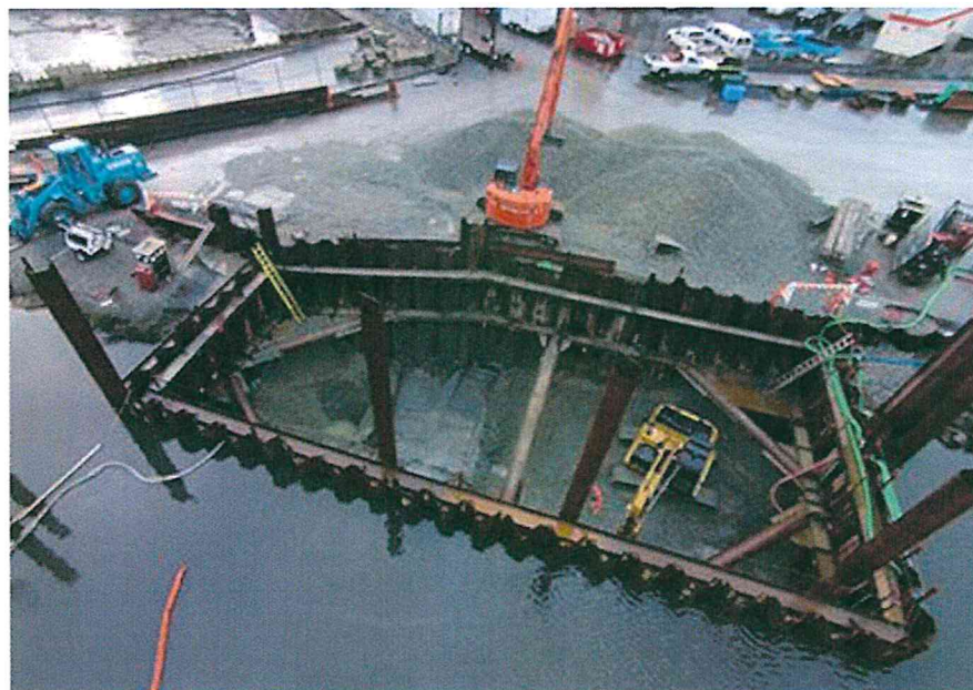
Figure 5: Cofferdam Construction (sourced from: www.qmenv.com )
