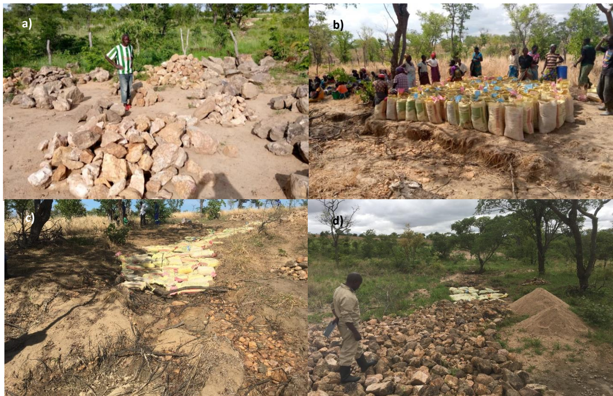
Figure 7: a) Dam committee vice-chairperson standing next to rock collected by the community; b) sand-filled sacs to be placed in rill erosion; c) placed sand-filled sacs; d) Maambo (MOA) assessing rock placement atop sand-filled sacs
