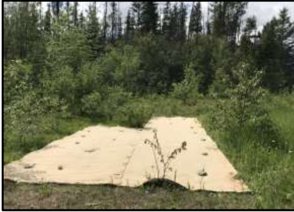
Figure 5. Photo of hemp matting, staked and weighted with rocks
