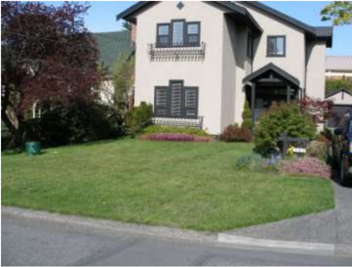
Before renovation (April 2011)
