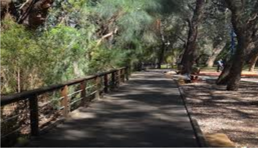
Figure 7: Riverside boardwalk at Centennial Pioneer Park, Perth, Australia. An example of elevated boardwalk with one side handrail/guardrail on swamp side that would serve to protect against erosion, compaction, minimize human and dog intrusion and would allow amphibian migration (missing plexiglass). From Weekend Notes. G. Adams, 2013, Retrieved November http://www.weekendnotes.com/treetop-walk-riverside-boardwalk-centennial-pioneer-park/
