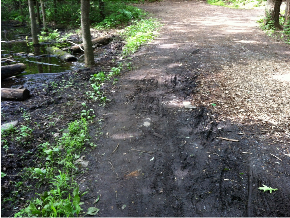
Figure C1: Recreational and maintenance vehicle trail bordering in (too) close proximity to the east side of the swamp demonstrating significant signs of erosion, soil compaction and ruts and invasive species. [Photograph], by Kerri Landry (author), 2013.
