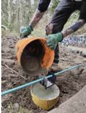
Figure 26. Evan Cline pouring concrete for the fence posts
