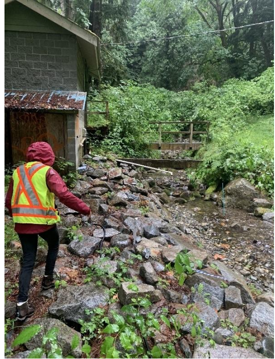
Figure B2: Site 1, Facing Northeast
