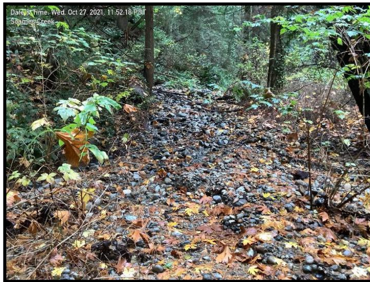
Photo 2: The area of slope/bank failure in a Soames Creek tributary, located above the well building. The result is significant large wood debris and bedload input into Soames Creek mainstem, resulting in the channel avulsing (changing directions) and forming numerous debris jams.
