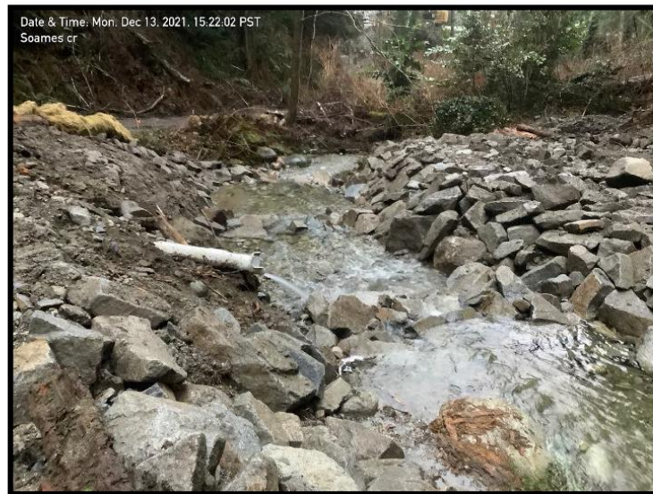
Photo 5: Finished channel above and below the SCRD well building. The channel, along the slope on the right bank was armoured and a series of weirs build within the channel to reduce the grade and help dissipate stream energy.
