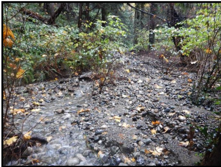
Photo 1: Soames Creek at the SCRD well building. An upslope failure (October) and extreme highwater events (November) has resulted in the creek channel infilling and the channel avulsing, eroding the area around the well building creating unstable and unsafe conditions for the structure.
