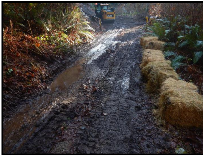
Photo 3: The main access road to be used for the reconstruction/excavation of the creek channel. The roads presents the greatest risk for sediment input. The access road was lined with hay bales and eventually capped. Once complete the hay was broken apart and used to cover the road to limit the possibility of sediment transport during poor weather.
