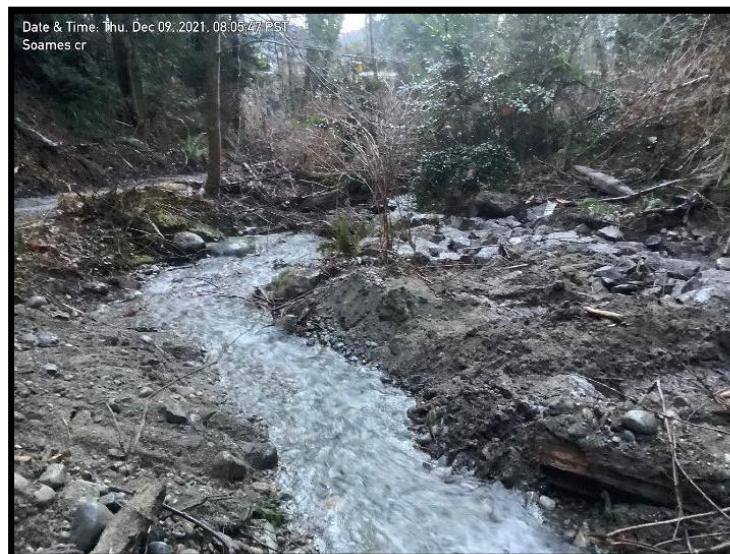
Photo 4: Newly excavated channel. This is the original channel that was infilled following the upstream “events”. The works and engineering design required re-establishing the original channel, located away from the building and infrastructure.
