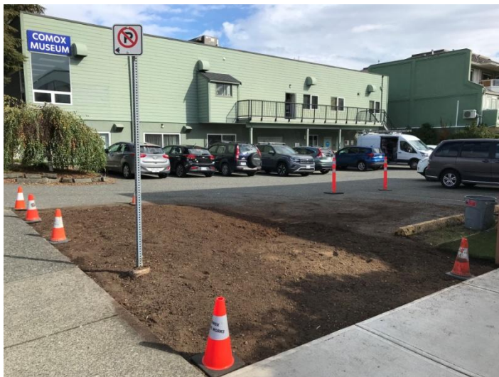
October 9, 2024 –The existing shrubs, their roots and a bark mulch layer were removed by the Town using a small skidsteer.
