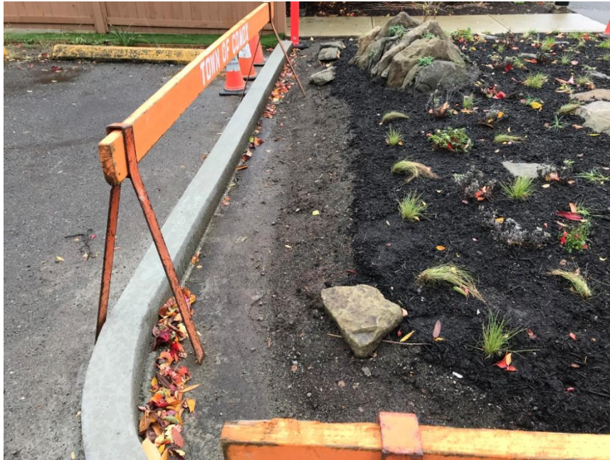
October 27, 2024 – Curbs installed. Note that the asphalt extends under the curb into the bed by as much as 20 cm in some areas.
