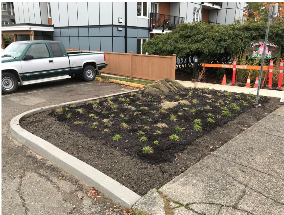
November 2, 2024 – backfill remaining soil mixture to curb
