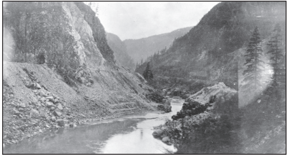
Clearing Hell's Gate slide, City of Vancouver archives.
