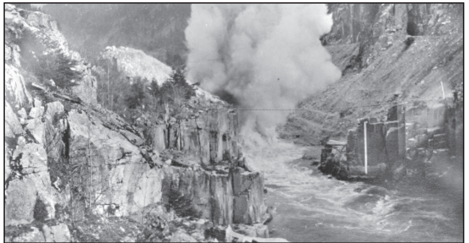
Clearing Hell's Gate Rockslide, Fraser River ca.1916, Vancouver Public Library.
