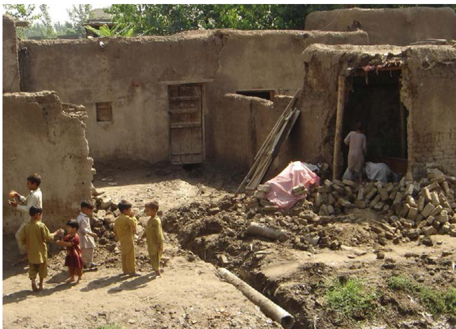
Disrepair in Afghan IDP Camp near Peshawar 2010, author photo
