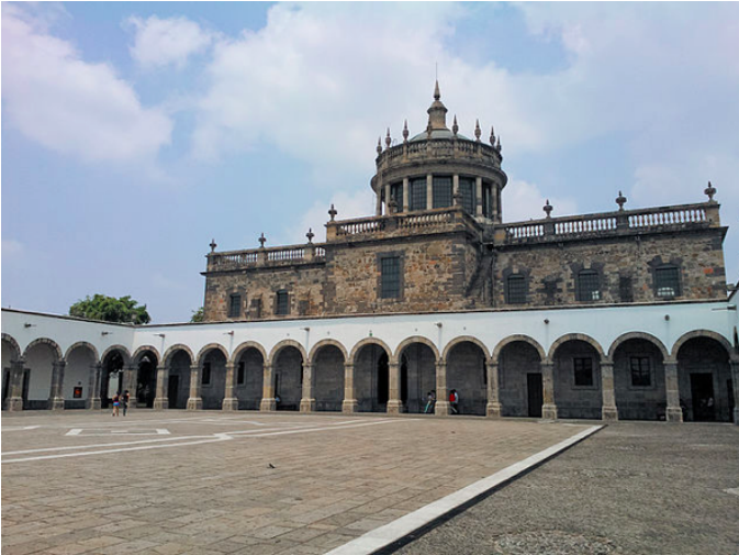
Figure 3. Tolsá, Manuel. Hospicio Cabañas. 1791-1829, Guadalajara, Mexico. View of main courtyard and chapel dome.
